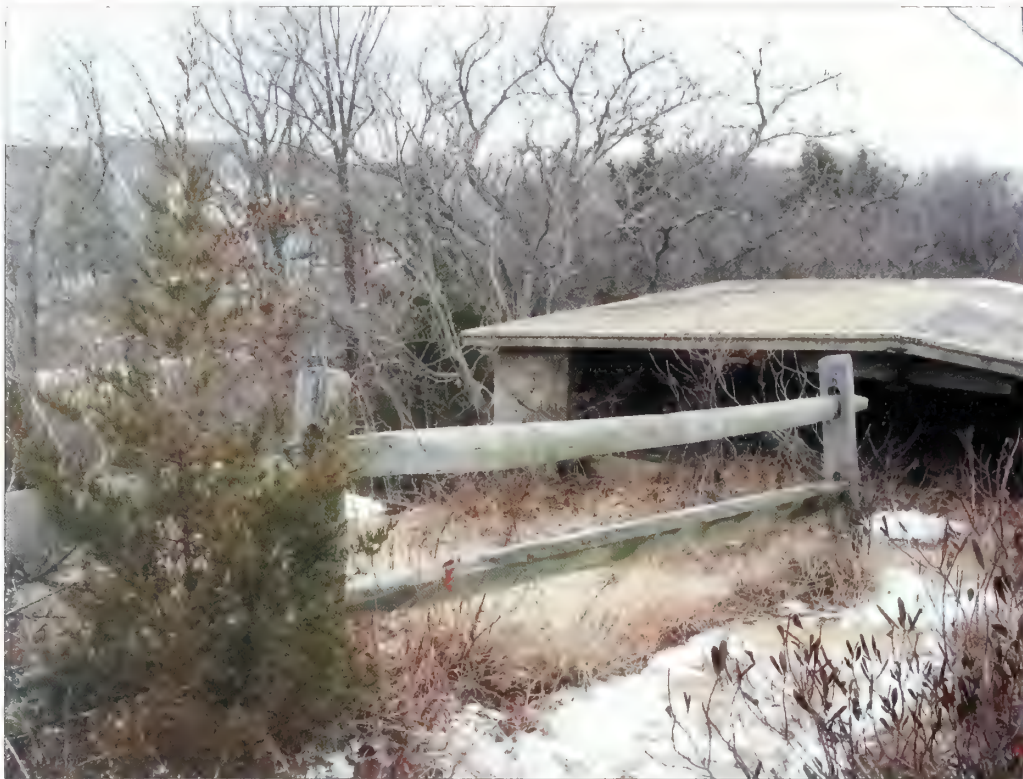
Figure 3.11. View looking northwest at Battery Engle (CRF Station Peck). The concrete coincidence range finder station (CRF) constructed on top of Battery Engle is located west of Battery Peck and features a low-pitched concrete roof. The structure appears in fair condition with some minor efflorescence visible on the roof (Olmsted Center, January 2009).
